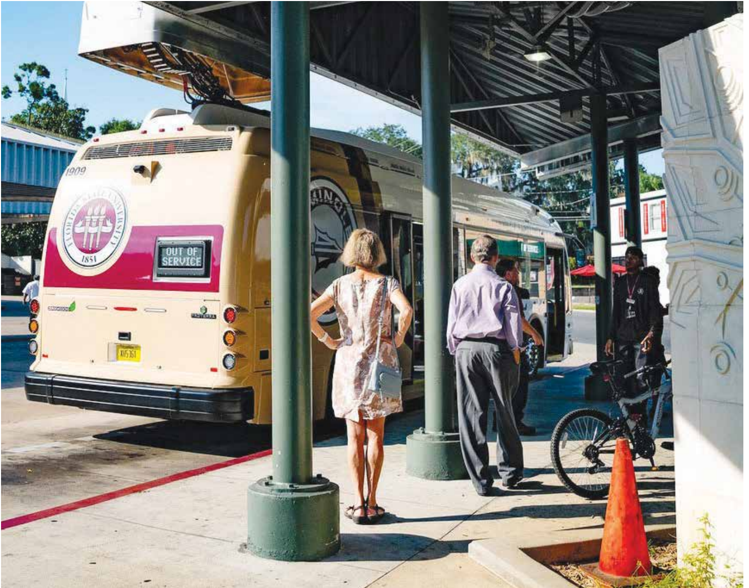
An example of StarMetro's electric bus charging infrastructure
